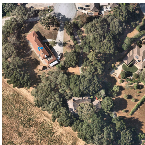
Figure 11: Two neighboring homes that were in the 2020 River Fire.
