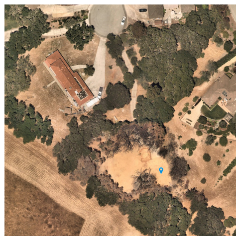
Figure 13: The aftermath of the wildfire that destroyed the bottom right building (blue marker) in Figure 11 & 12.
